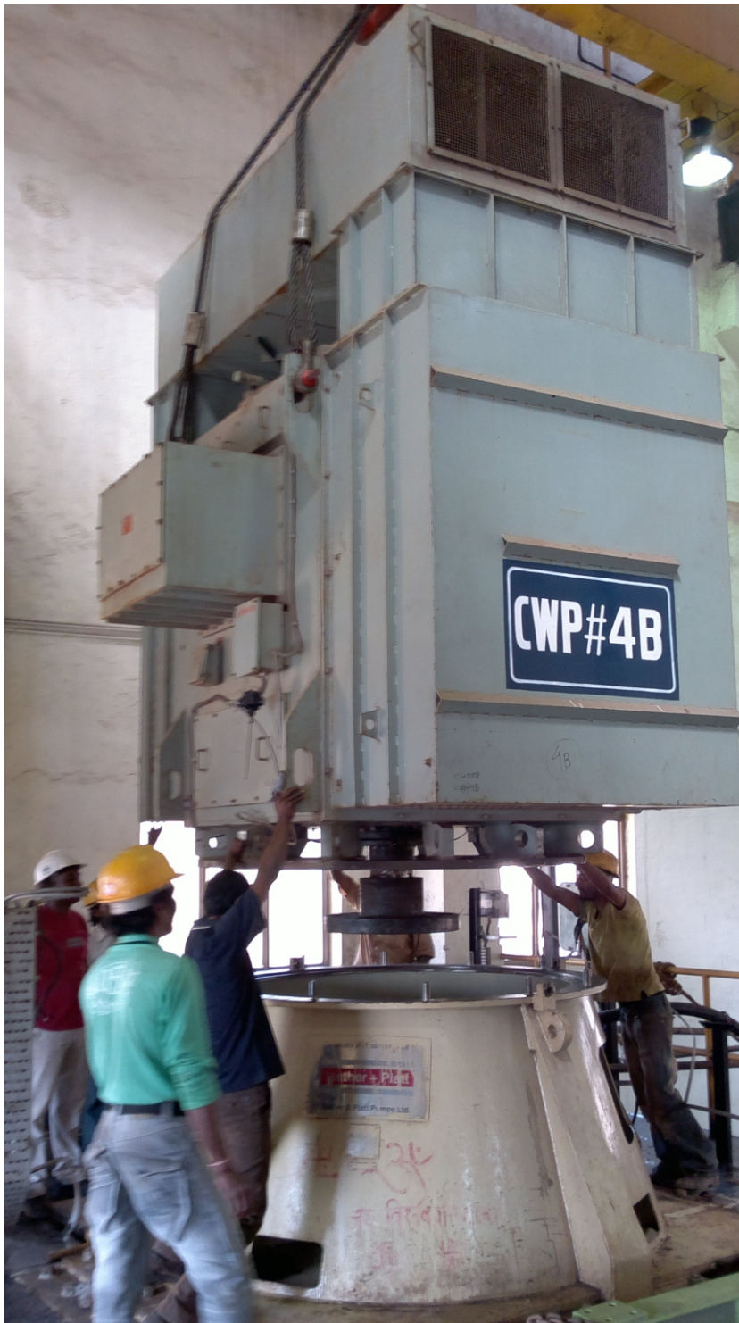
CW Pump overhauling
