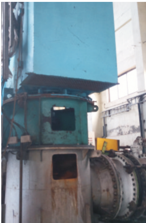
Sea Water Pump Overhauling
